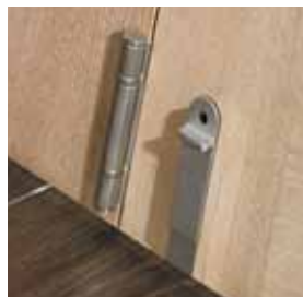
DROP BOLT / LIFT BOLT
